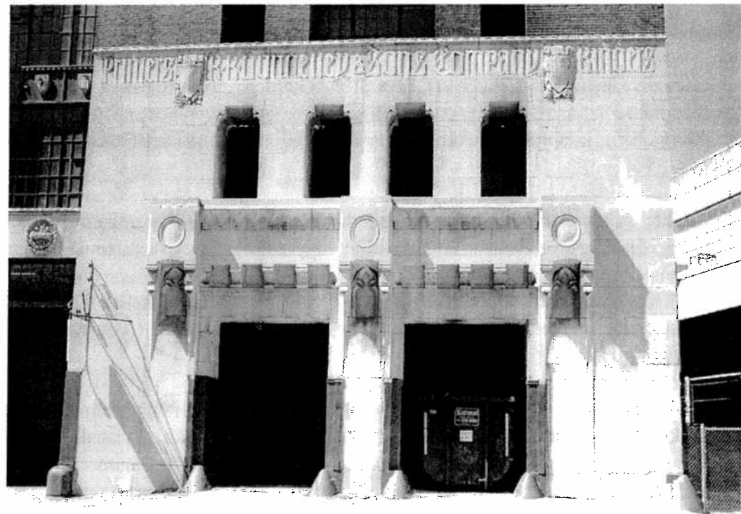
Right: The Calumet Plant's southeast tower, built in 1929 and designed by Charles Klauder after the death of Howard Van Doren Shaw, has a decided vertical emphasis. Below: The tower's base is clad with gray limestone and detailed with Gothic-style ornament, including the Donnelley company's name in Gothic script.
